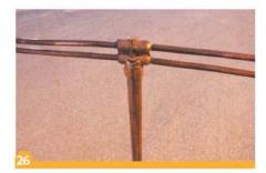
Welded earthing conductors and earthing electrod.
